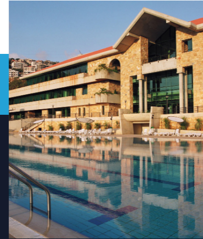
CLUB JEITA COUNTRY CLUB - LEBANON SCOPE: Electrical Installations, Electrical Power Plant – Transformers, Generators, Main & Sub- istribution Panel Boards. Mechanical Installations.
