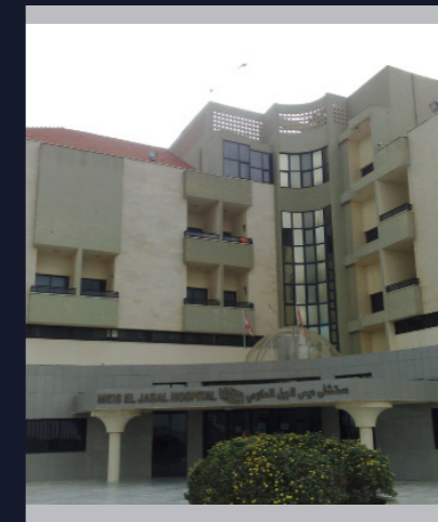
HOSPITAL MEISS AL JABAL HOSPITAL - LEBANON Complete Supply & Installation of all Electrical & Mechanical Systems in a local Hospital in Southern Lebanon (five operating rooms).
