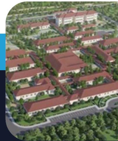
HOSPITAL KUMASI 250 BED REGIONAL HOSPITAL-GHANA SCOPE: ELECTRICAL WORKS ,POWER STATION, LOW CURRENT, VOIP
