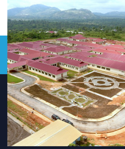
HOSPITAL KONONGO 60 BED DISTRICT HOSPITAL-GHANA SCOPE: HVAC - CHILLED WATER SYSTEM AND ELECTRICAL WORKS
