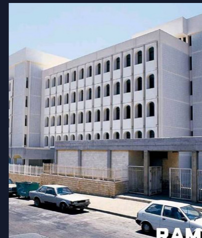
SCHOOL BIR HASSAN SCHOOL - LEBANON SCOPE: Electrical Power Plant – Transformers, Generators, Main & Sub- Distribution Panel Boards. Heating, Ventilation & Air Conditioning, Sewage, Fire Fighting, Rainwater, Drainage & Liquified Petroleum & Gas System.
