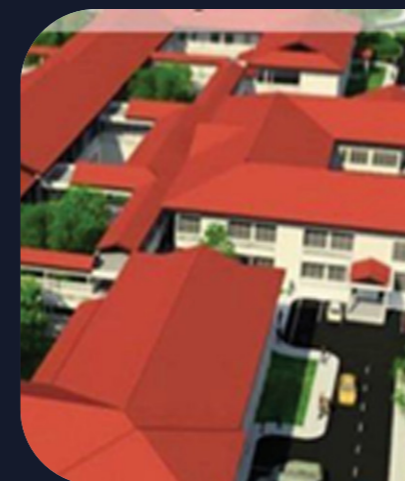
HOSPITAL SALAGA 60 BED DISTRICT HOSPITAL-GHANA SCOPE: ELECTRICAL WORKS ,POWER STATION, LOW CURRENT, VOIP, PLUMBING , FIRE FIGHTING & HVAC
