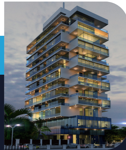
HOTEL OXFORD NO.01- ACCRA-GHANA SCOPE: ELECTRICAL WORKS ,POWER STATION, LOW CURRENT, VOIP, PLUMBING, FIRE FIGHTING, HVAC, BMS, LIFTS ..
